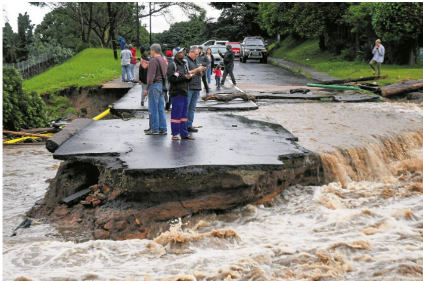
Figure 2. Harm to roads due to spring 2022 floods in the coastal area.
