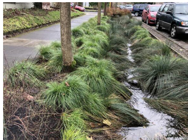
Figure 5. Green street planters.
