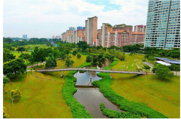
Figure 4. Kallang River at Bishan-Ang Mo Kio Park.
