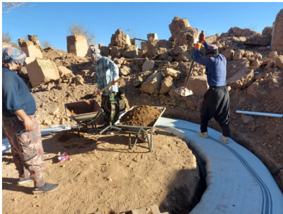
Figure 3. Execution of foundation and wall of Super Adobe shelter in Sanjab, Herat.
